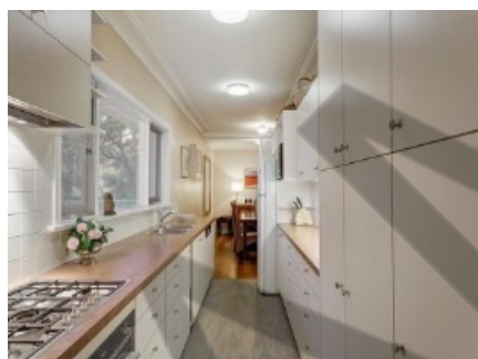
Rangehood exhausts into roof space
