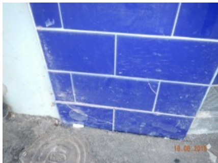
Building on front boundary - No access
